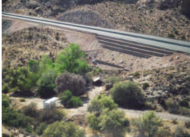
Hilfiker Wall Constructed on SR 68
