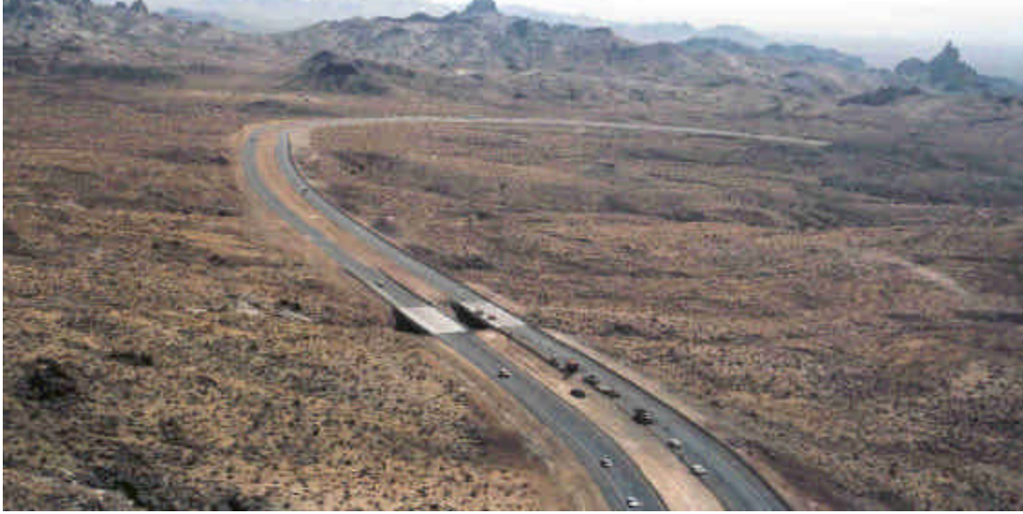
Construction of SR 68
