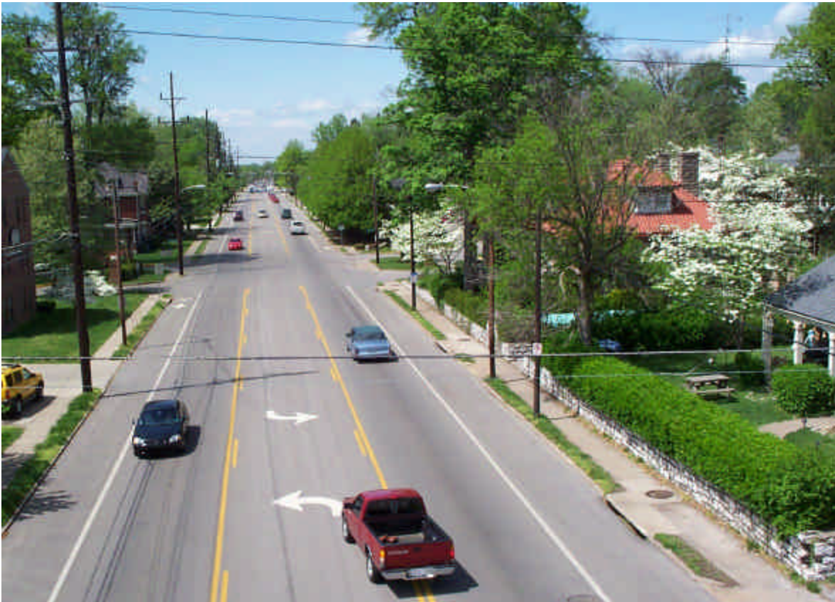
Figure 4. Current conditions (east-bound view)
