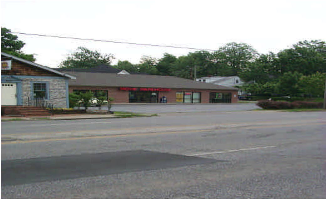
Figure 1. Existing conditions (4-lane with narrow median)
