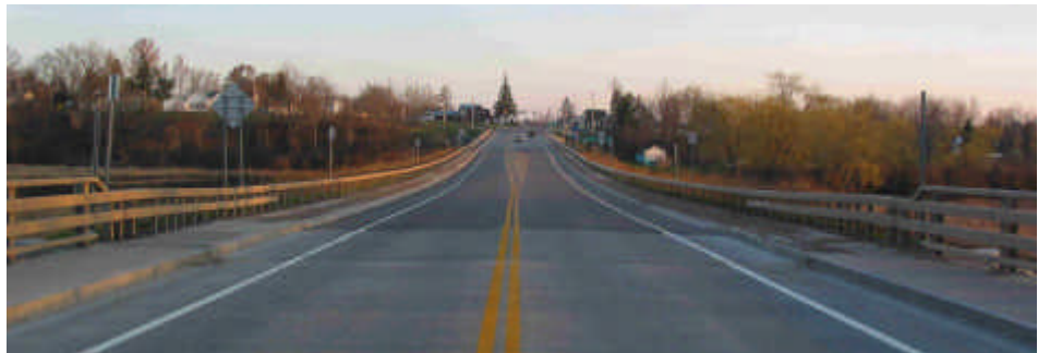
Figure 7: Salmon River Bridge (looking South)
