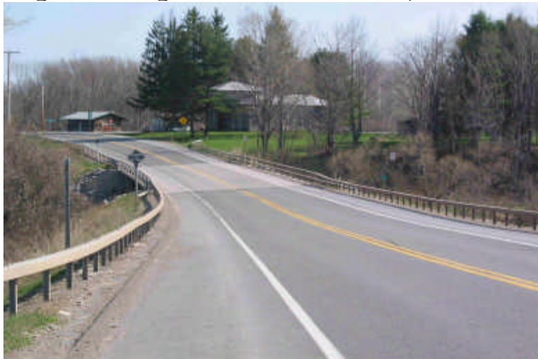
Figure 5: Bridge over Grindstone Creek (south of Port Ontario)
