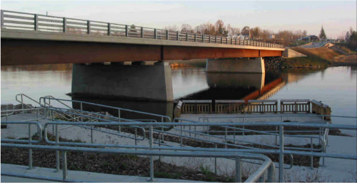
Figure 8: Completed Salmon River Bridges
